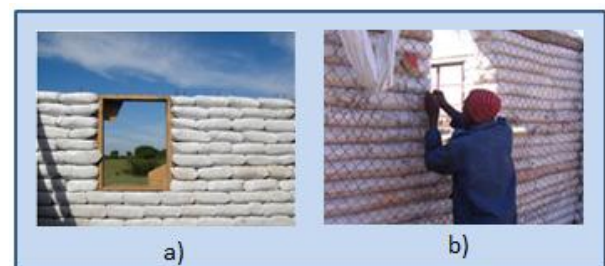
Figure 2: (a) Earth bag wall construction with bags filled with earth and laid in courses like bricks (b) Superadobe earth bag wall construction tied with parallel strands of barbed wire are laid between courses to act as a kind of mortar.
